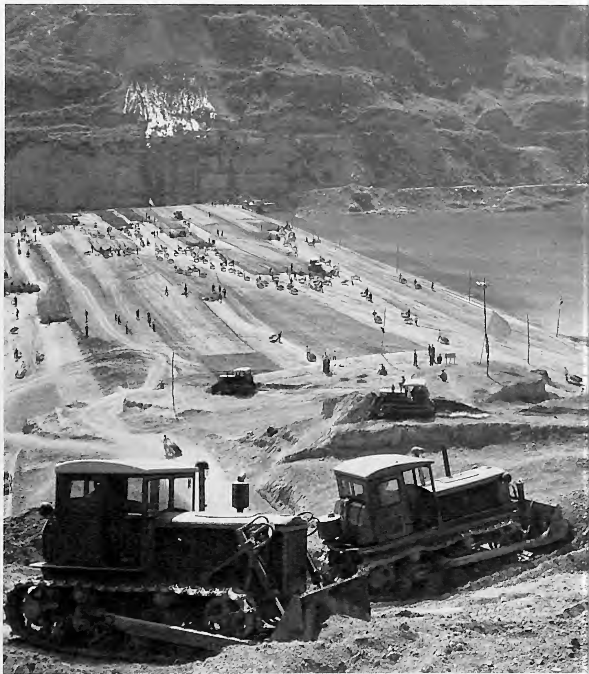
Capital construction on the farmland. By Huang Chi-hsien
